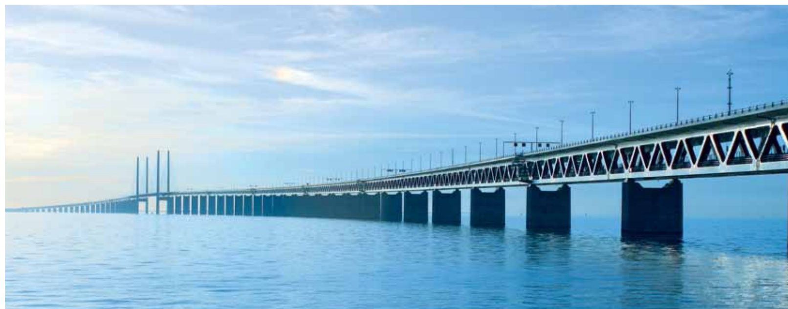
Connecting Denmark and Sweden since July 2001: the 7.845 km long Öresund Bridge.
