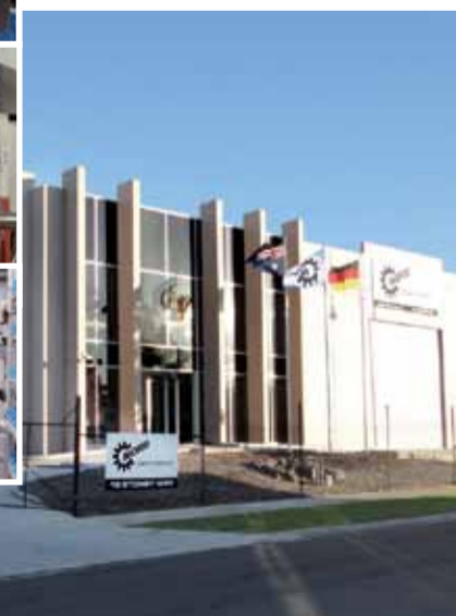
There was much to see in the ultra-modern assembly and service facilities of NORD Australia.
