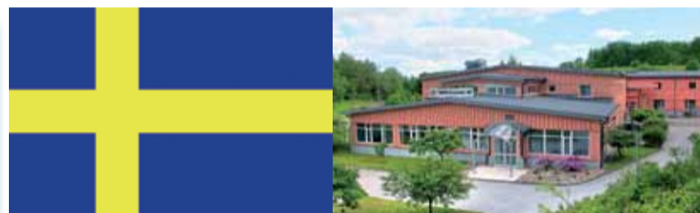
NORD DRIVESYSTEMS AB headquarters, Upplands Väsby, Sweden
