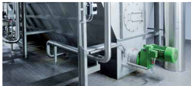
A parallel shaft gear is used to drive the screw conveyor and to remove the spent grain.
